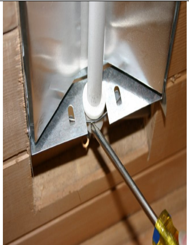
10. Remove spring clip shown here
