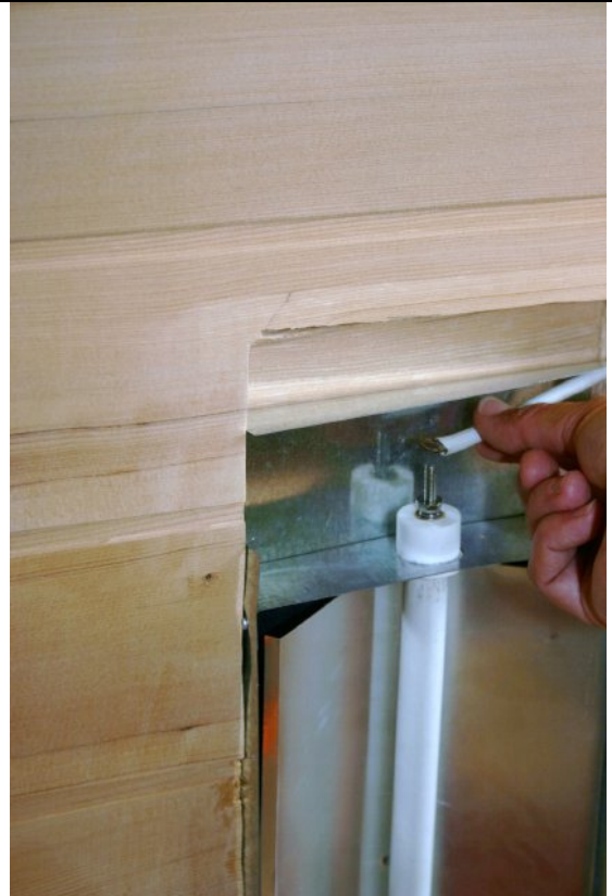
8. Remove wire from top of heater
