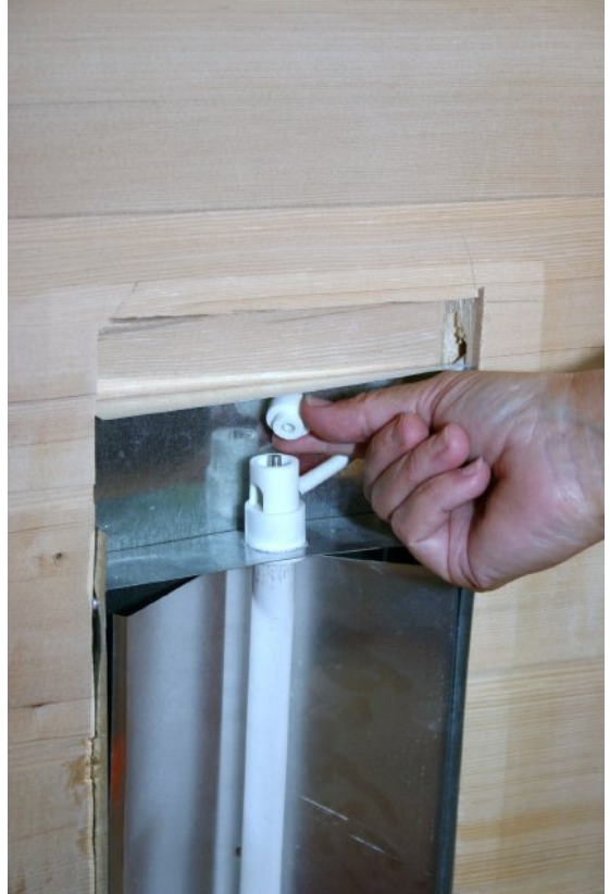
4. Ceramic cap shown removed
