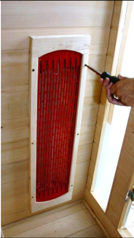
1. Remove screws from heater guard
