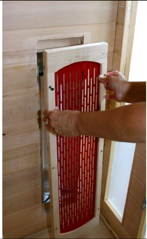
2. Remove heater guard
