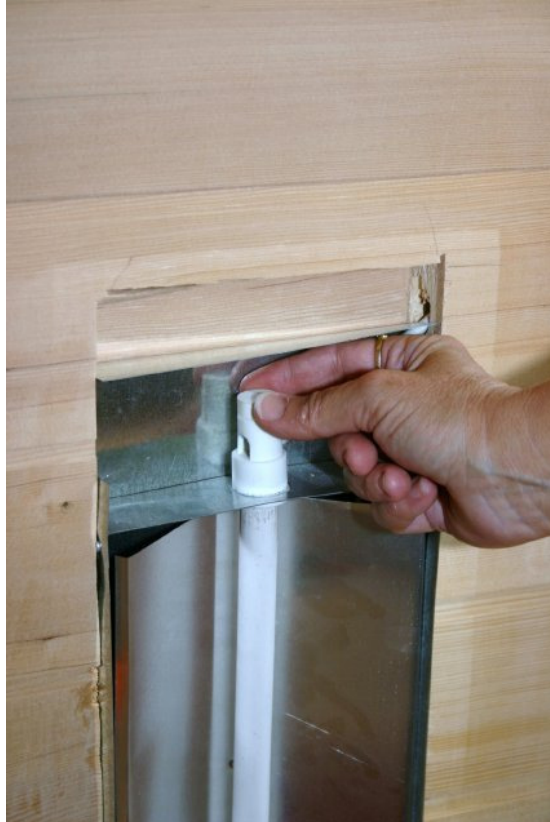
3. Unscrew ceramic cap from top
