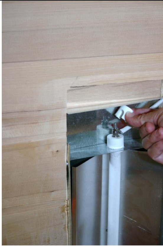
5. Remove ceramic wire guard
