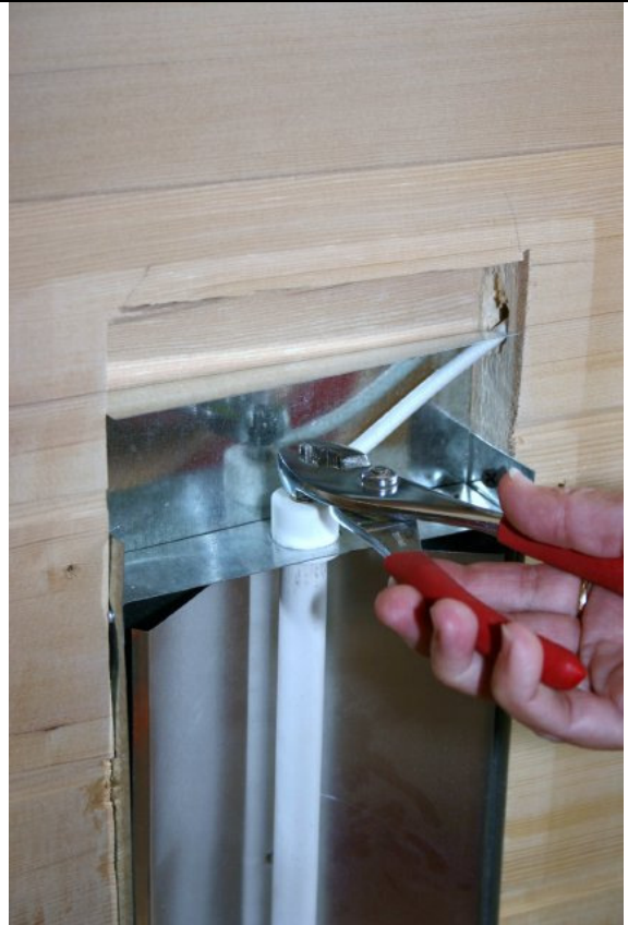
6. Use pliers or small wrench to remove nut.
