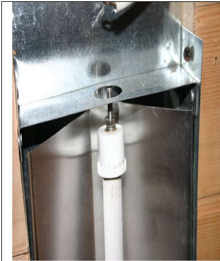
13. Drop heater down through top hole
