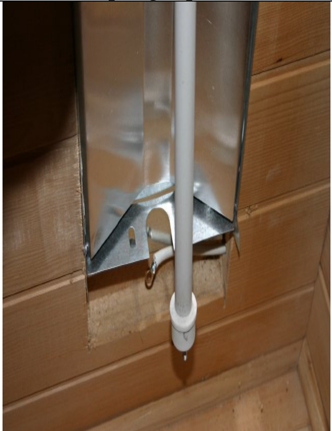
12. Pull ceramic heat forward at bottom.
